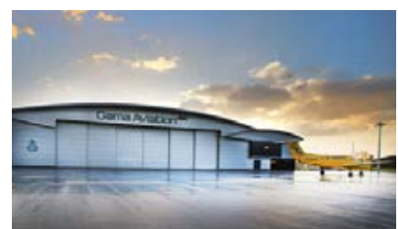
Ground lease to Gama Aviation, Glasgow Airport
